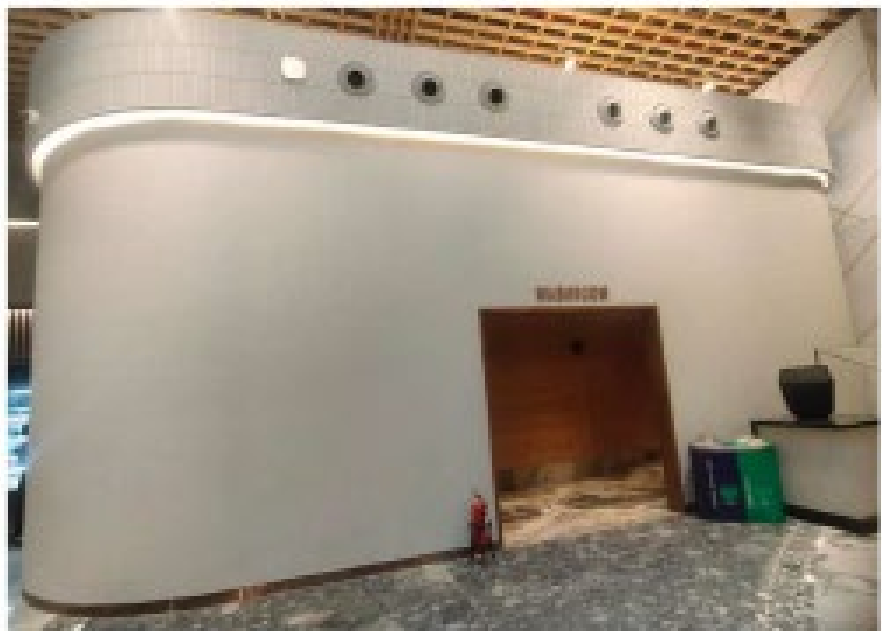
Bangalore International airport, Terminal 2
